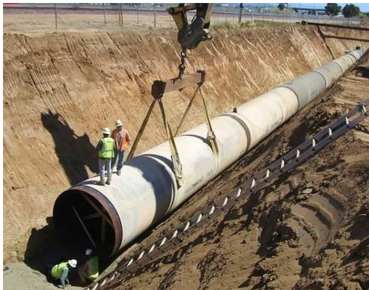
Open-Cut Trench Pipeline Construction – Representative Photo
